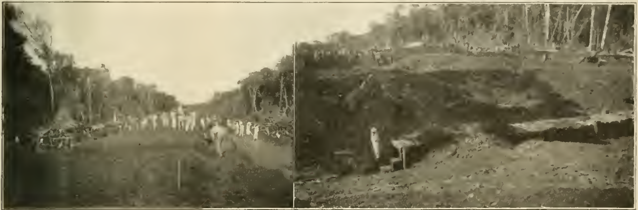
Grading for 20th mile.
